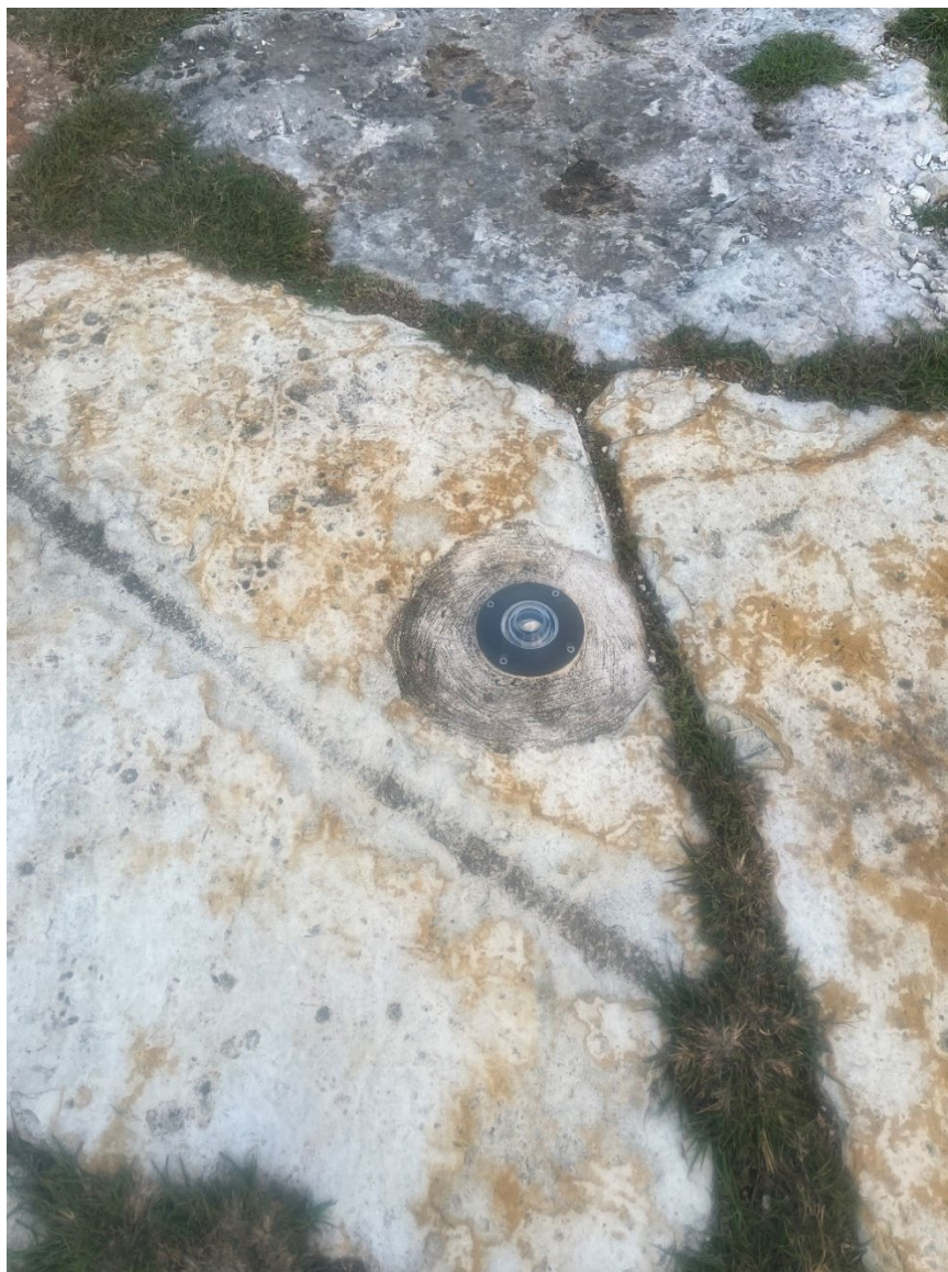
Photograph 8 - View of the private heliport lighting (courtesy of the Federal Aviation Administration)
