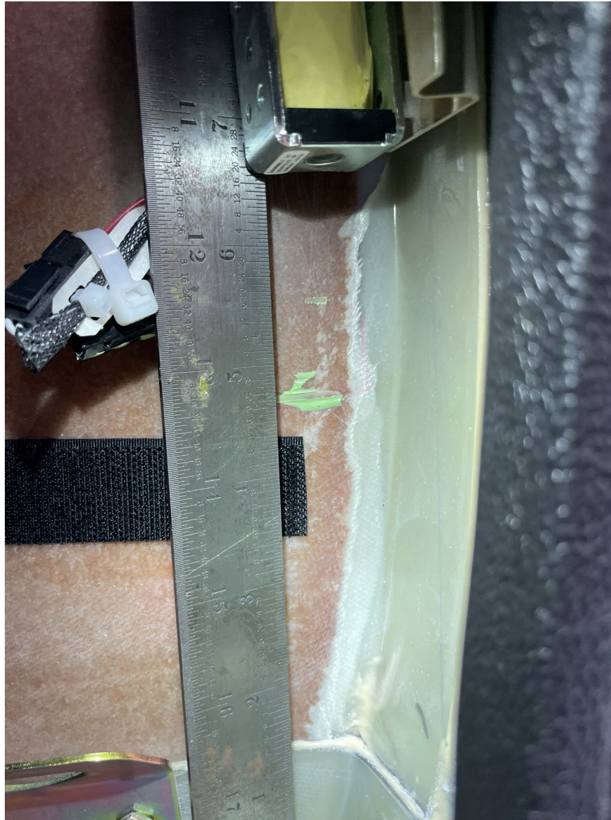
Photograph 2 - Delaminated Bulkhead (Courtesy of FAA)
