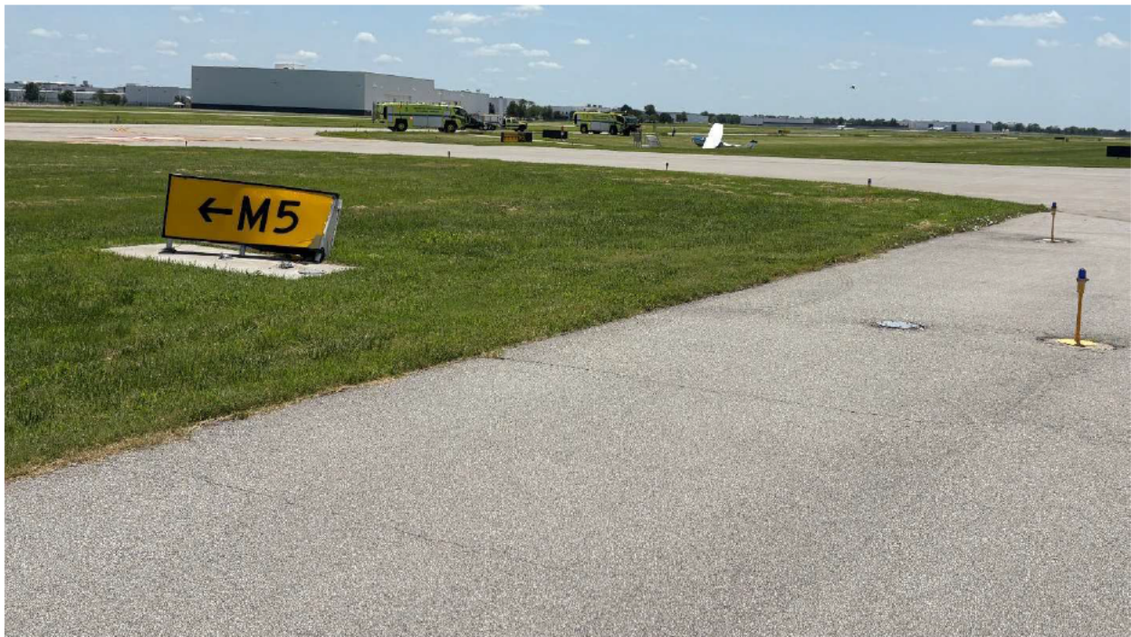
Photo view to south southeast. Damage to sign M5 pavement to the right is the edge pavement of runway 19L. Rescue trucks are parked facing west on taxiway M.
