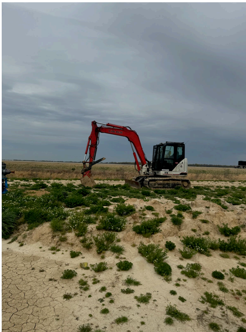
Photograph 2 - Excavator struck by accident airplane (Courtesy of Sheriff's Office)
