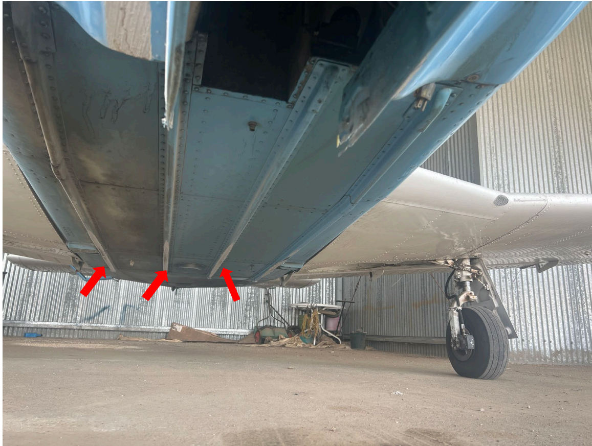
Photograph 2 - Damaged longerons on belly of airplane (Courtesy of FAA)
