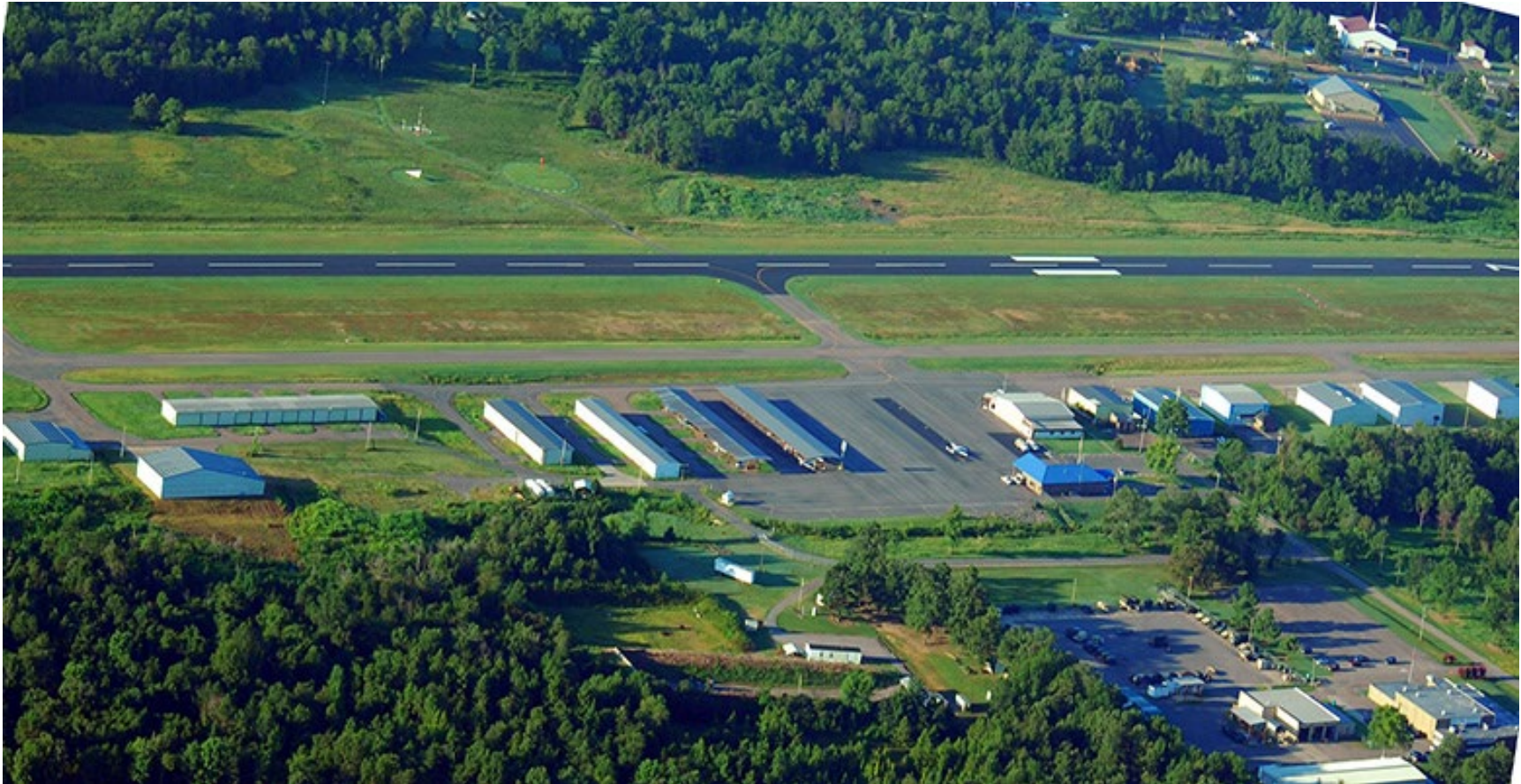
Photograph 2 - Aerial view of the accident airport, looking to the south (courtesy of the Russellville Regional Airport)
