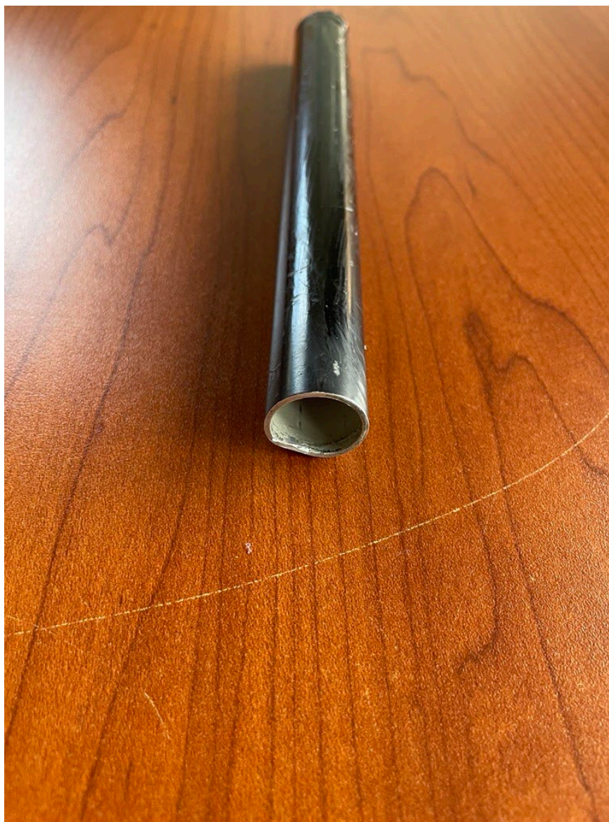
Photograph 2 - Separated Anchor Point (Courtesy of NTSB)
