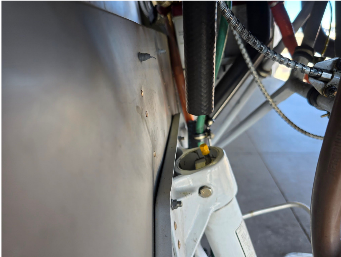
Photograph 1 - Firewall buckling (Courtesy of USAFA Aero Club)
