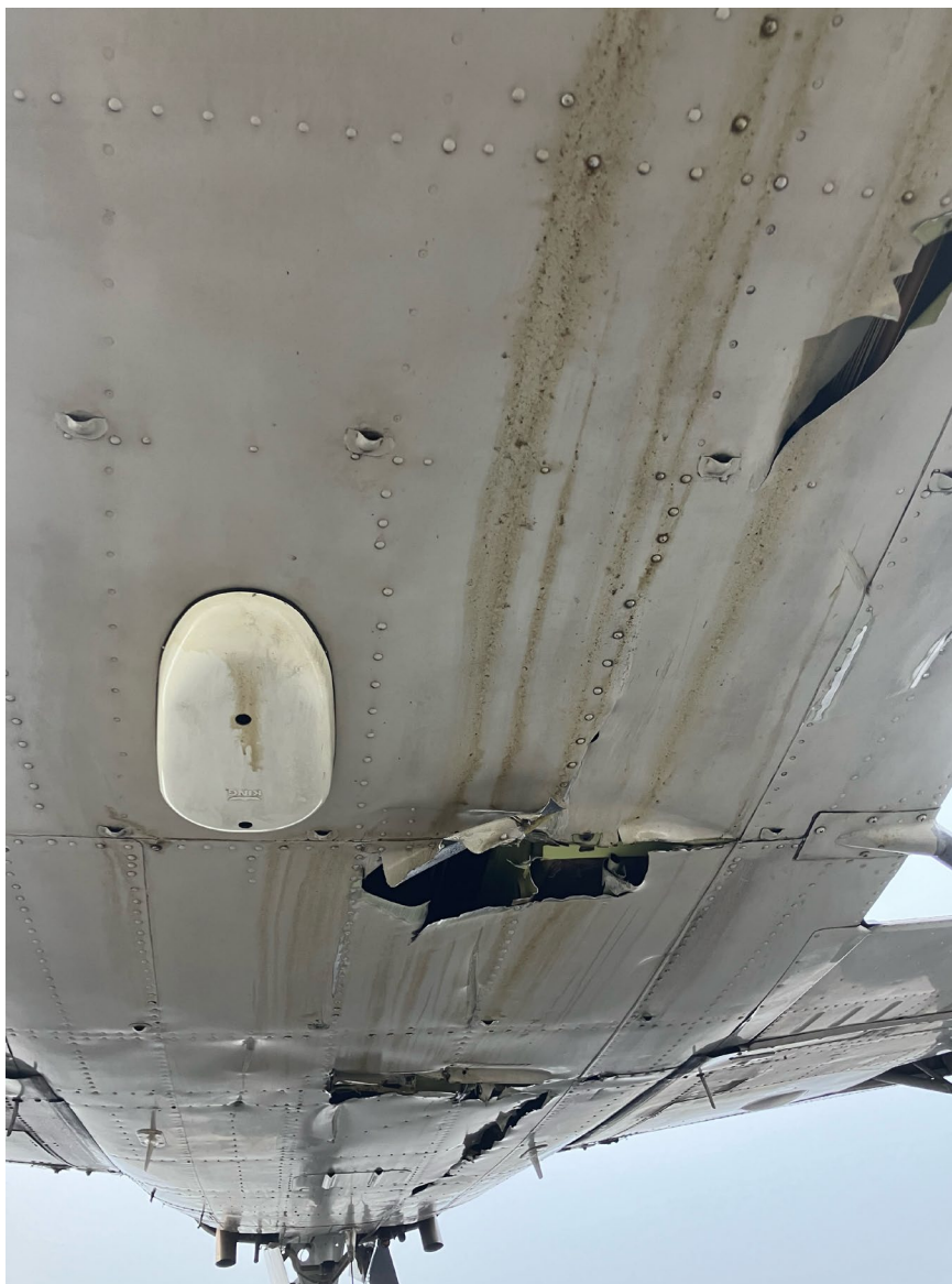
Photograph 2 - Underside of Fuselage (Courtesy of Airport Manager)
