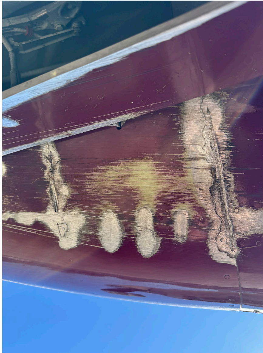
Photograph 2 –Fuselage damage (Courtesy of accident pilot)
