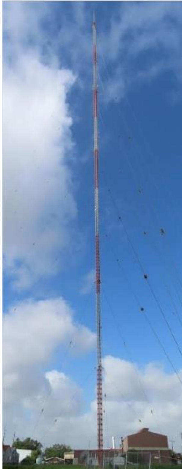
Figure 7. Image of the accident radio tower, courtesy of the owner.
