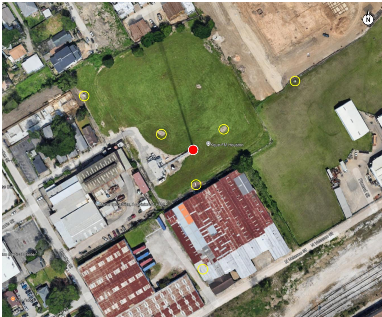
Figure 3. Image of the accident site. The red circle identifies the location of the radio tower. The yellow circles identify the anchoring points for the guy wires for the radio tower.
