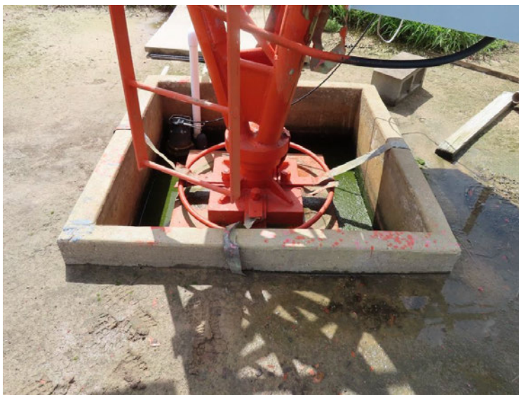
Tower Base Foundation
