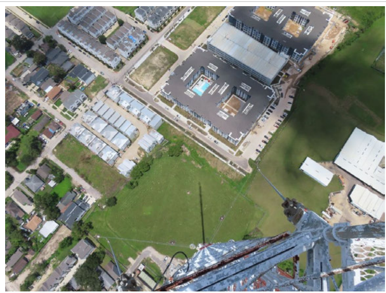
Aerial View of Tower Compound
