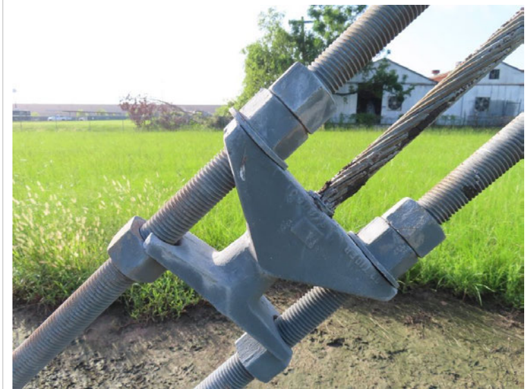
Guy Anchor Hardware (Typical)
