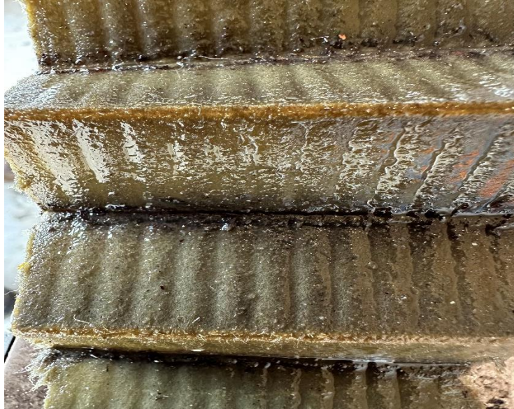
Debris in Oil Filter Element
