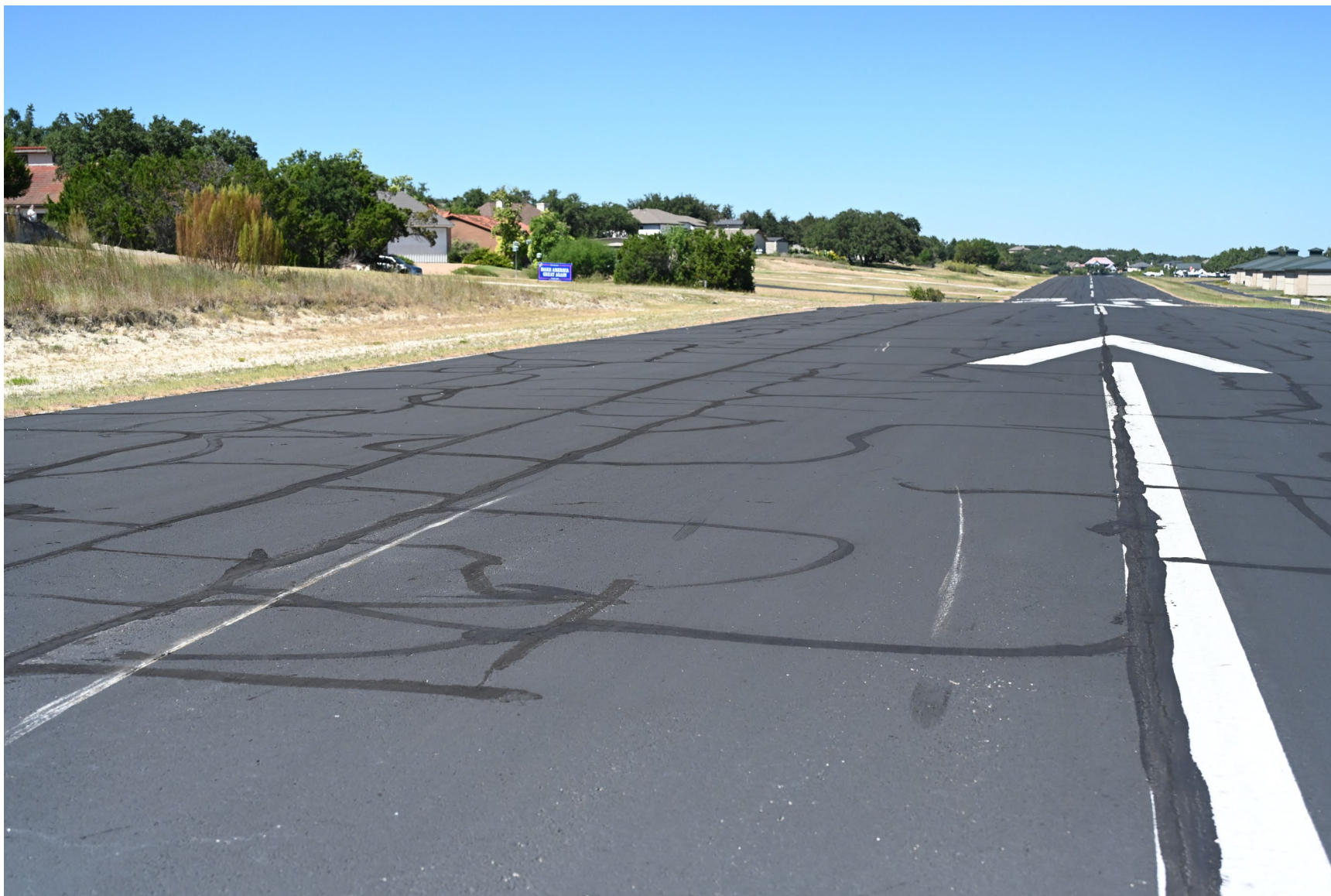
Photograph 2 - Impact marks on runway (Courtesy of Cirrus Aircraft)
