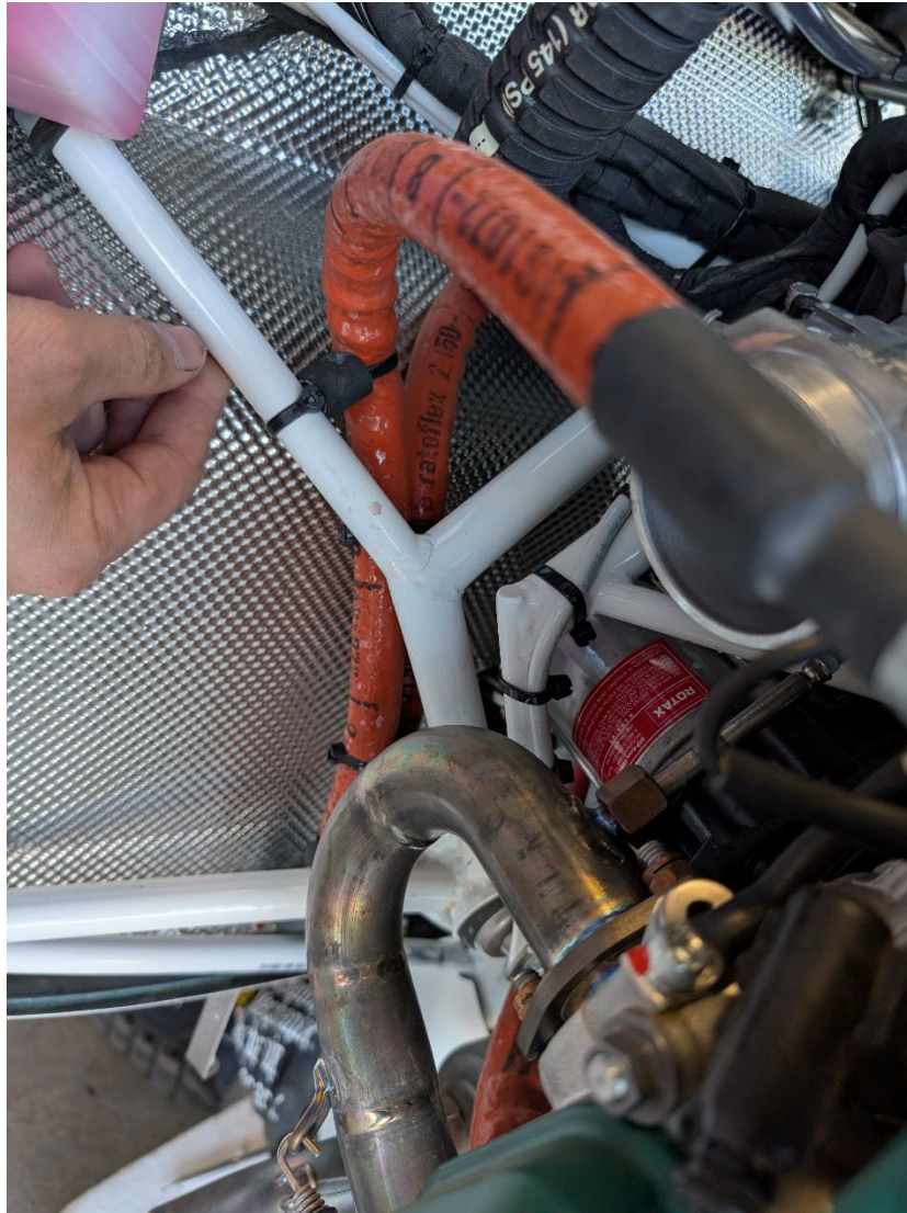
Photograph 2 - Engine mount (Courtesy of FAA)
