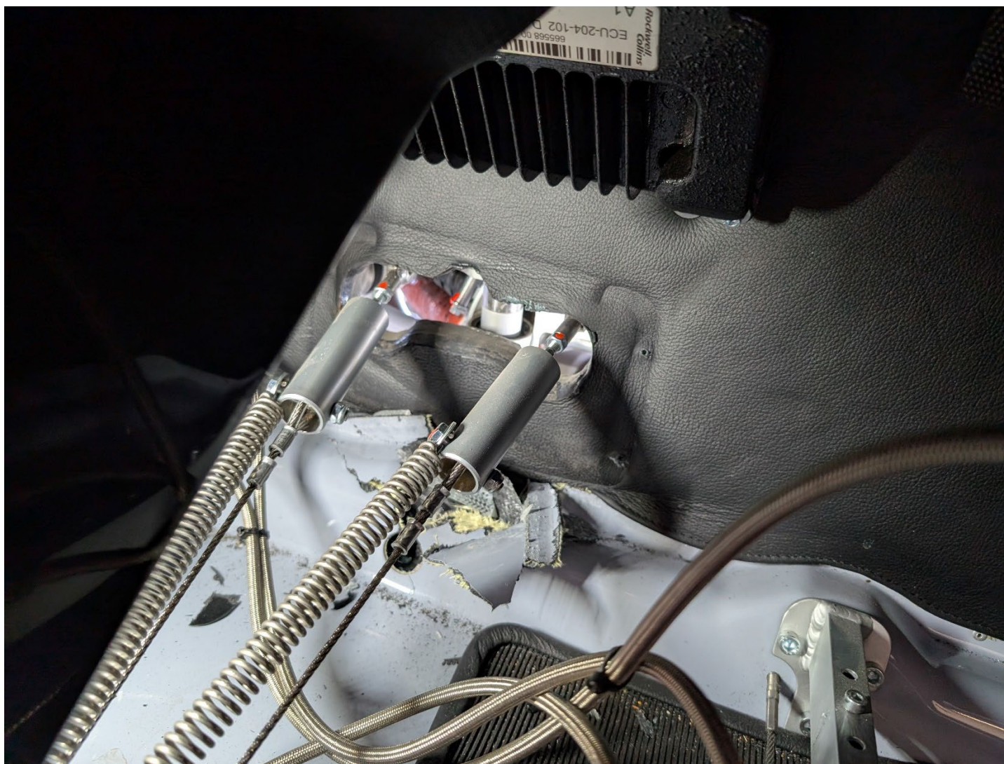
Photograph 3 - Composite damage (Courtesy of FAA)
