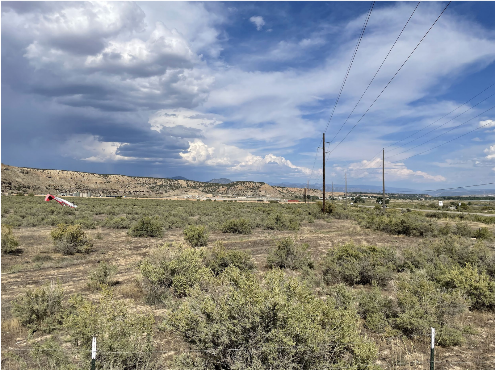
Photograph 1 - Accident site, power lines (Courtesy of private citizen)
