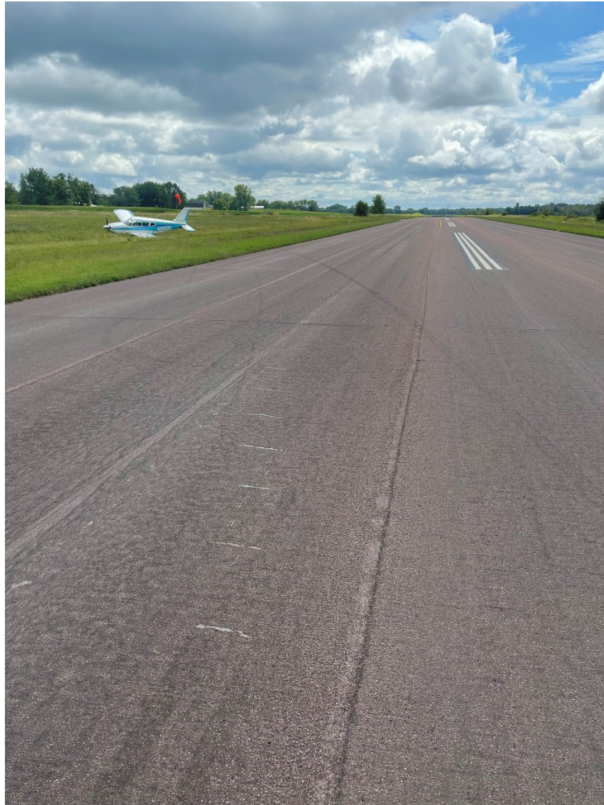
Photograph 4 - Ground scars on runway (Courtesy of FAA)
