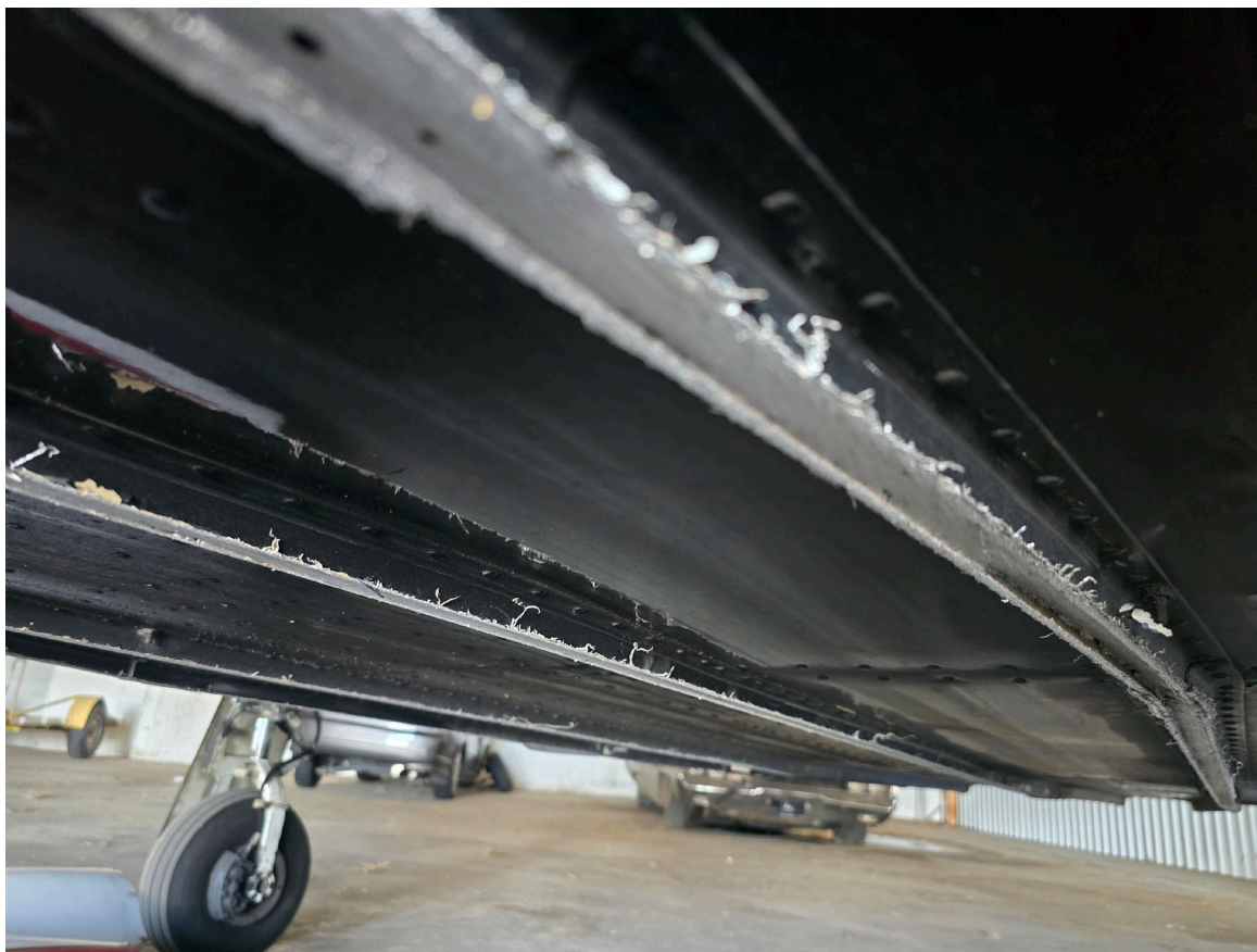
Photograph 2 - Damaged Longerons (Courtesy of Federal Aviation Administration)
