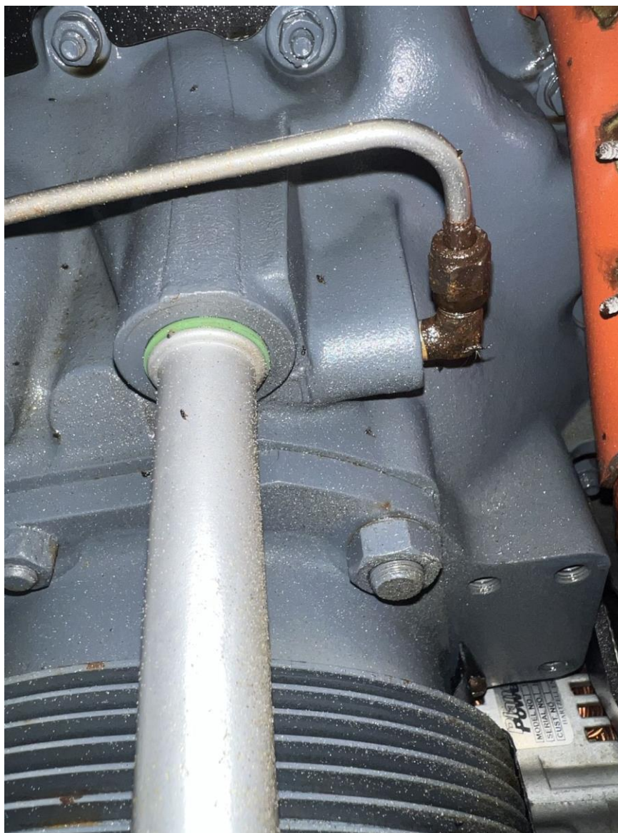
Photograph 8 - Engine Oil Pressure Line (Pilot Photo)
