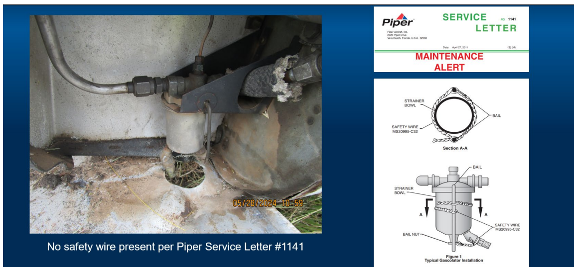
Figure 7 - Gascolator at Accident Site Prior to Removal by FAA
