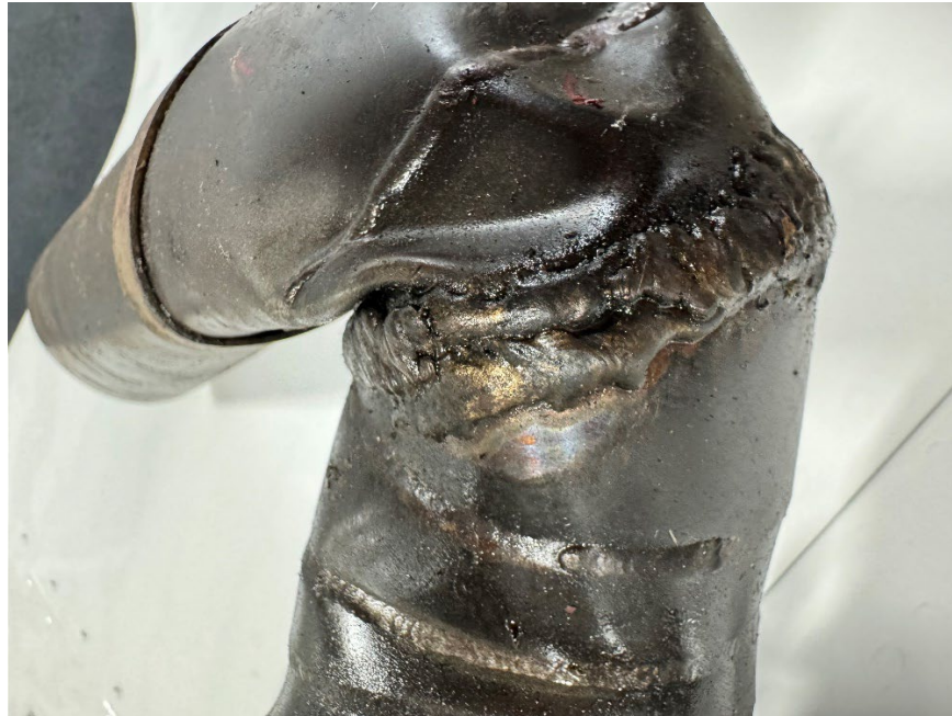
Figure 5. Exhaust repair weld
