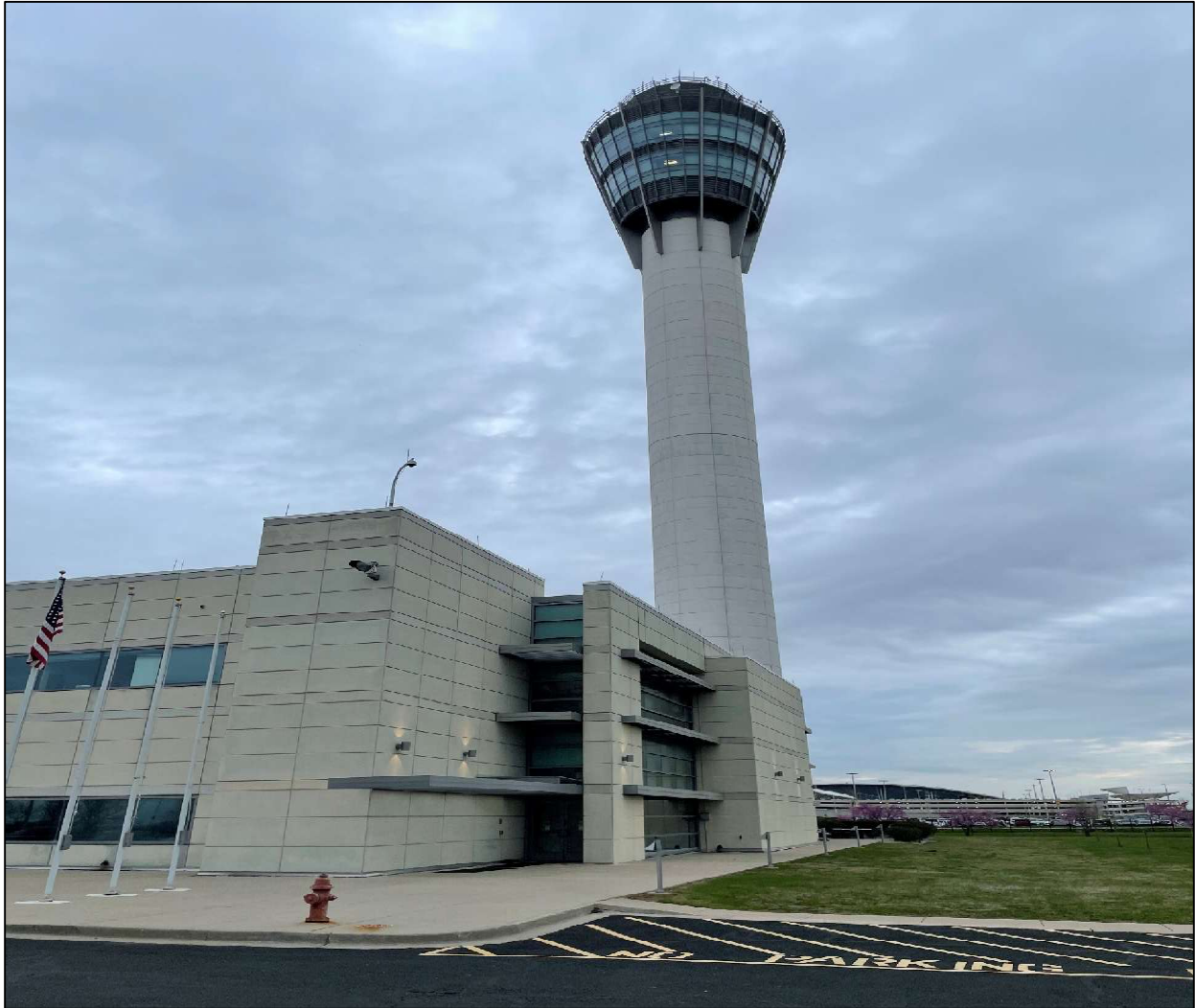
Figure 10. Photo of IND tower and TRACON at ground level taken by NTSB staff.
