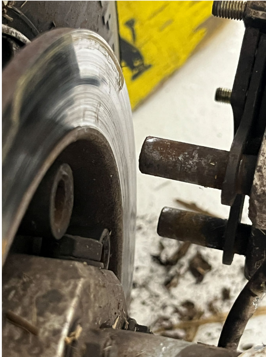
Photograph 3 - Corrosion noted to the anchor bolts (Courtesy of FAA)
