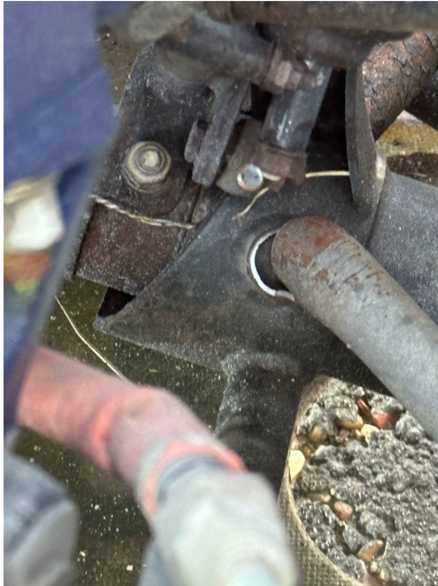
Photograph 5 - View of the fractured engine mount (Courtesy of Lubbock Aero)
