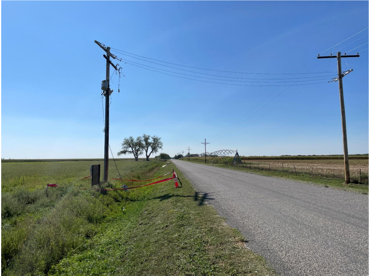
Figure 2 - Location of power pole as seen facing west along County Rd W.
