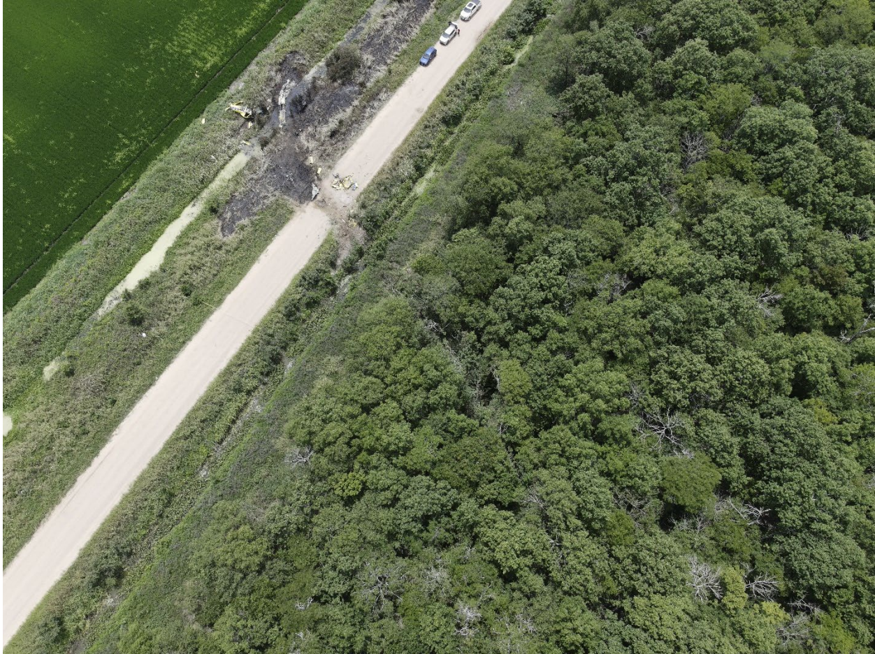
Figure 3. Aerial view of N6177J accident site.
