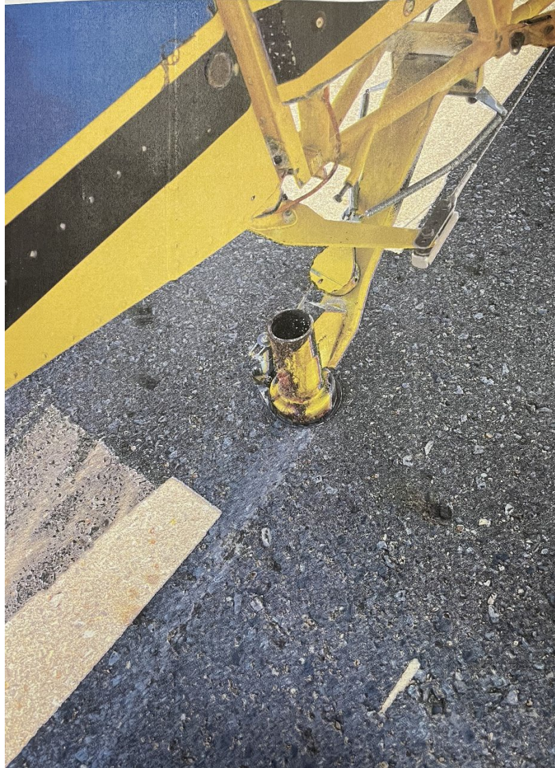
Photograph 3 - N795LA Missing Tail Wheel Assembly (Source: Operator)
