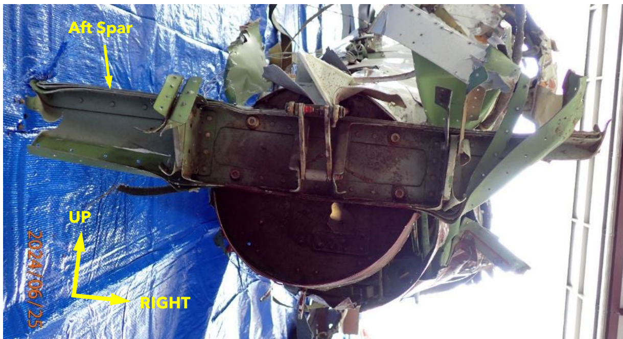
Figure 16. Horizontal stabilizer aft spar (NTSB photo)
