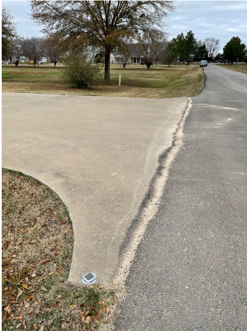
Photograph 7 - Driveway Deck Lights (NTSB IIC)
