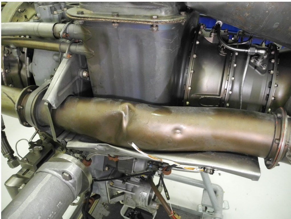
Photo 4 - Left Side Compressor Discharge Tube - Dents
