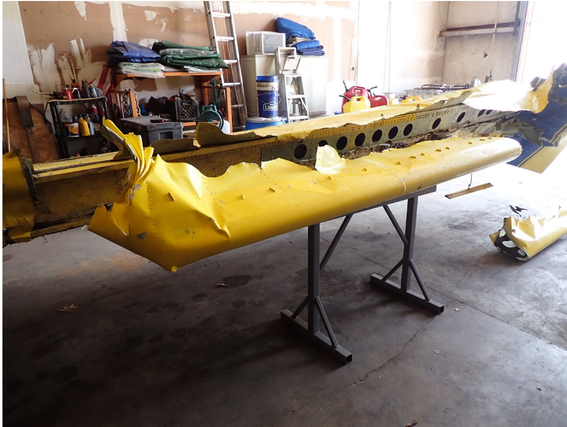
Photograph 4 - Left Wing Reconstruction (Courtesy of Air Tractor)
