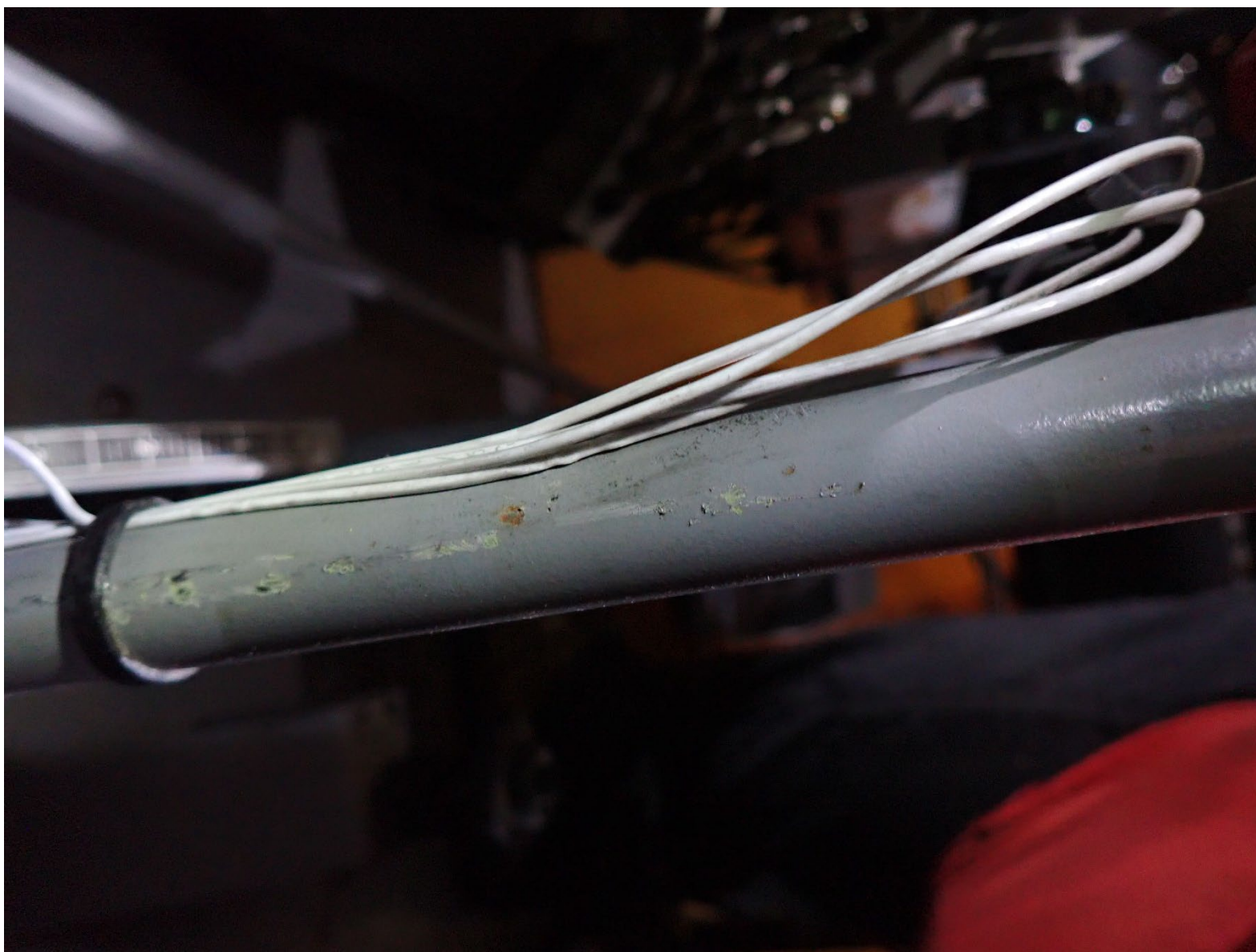
Photograph 9 - Spray valve pushrod scrapes (Courtesy of Air Tractor)
