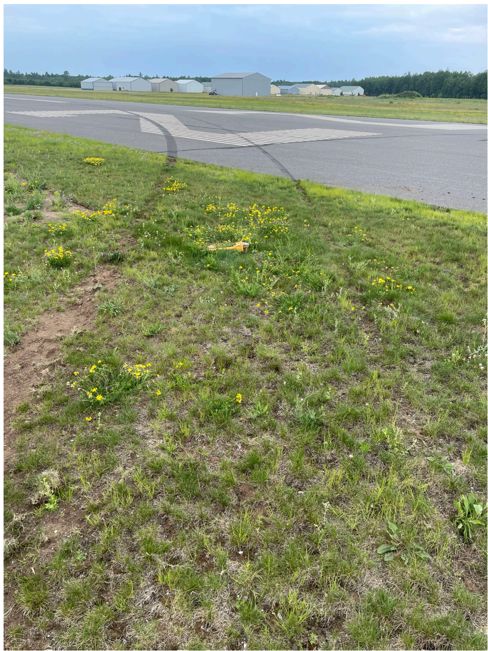
Photo 3 – Runway excursion tire marks (Source: FAA)
