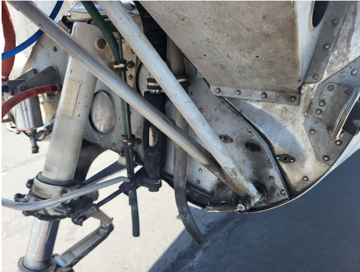
Photograph 1 - Bent and wrinkled airframe firewall (Courtesy of Operator)
