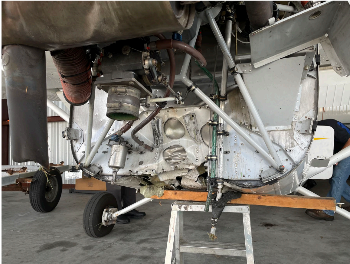
Photograph 2 - Wrinkled Underneath Side of Fuselage (Courtesy of FAA)
