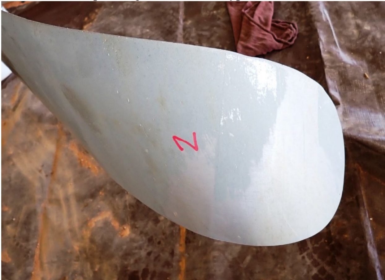
Figure 35: Tip damage on Blade #2, typical on all three blades
