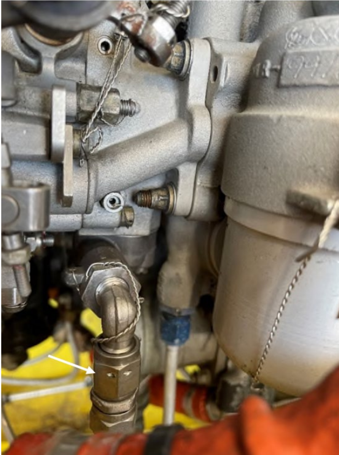
Figure 14 - P3 Fitting at FCU
