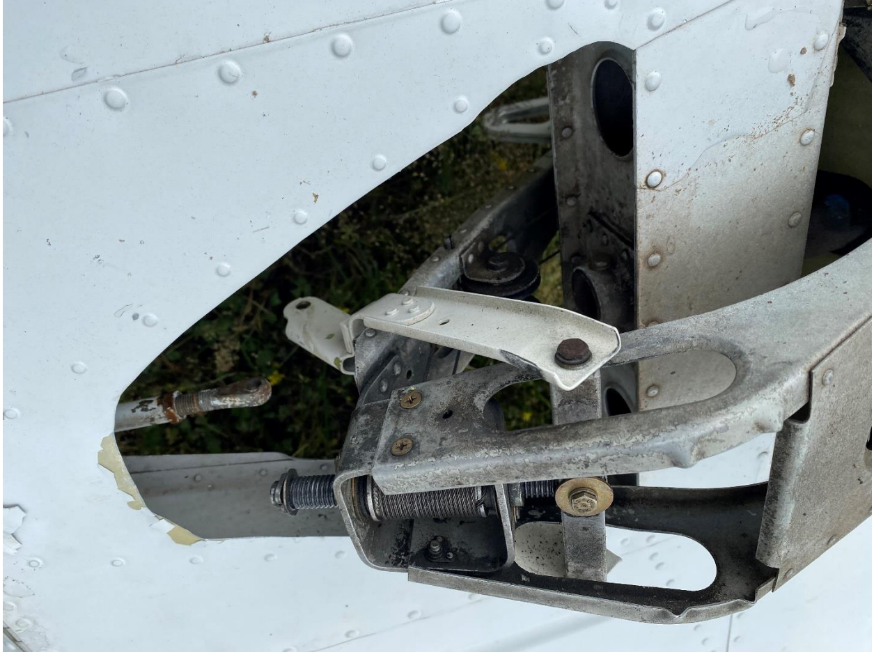
Photo 2: Trim Connection (Courtesy of the FAA)
