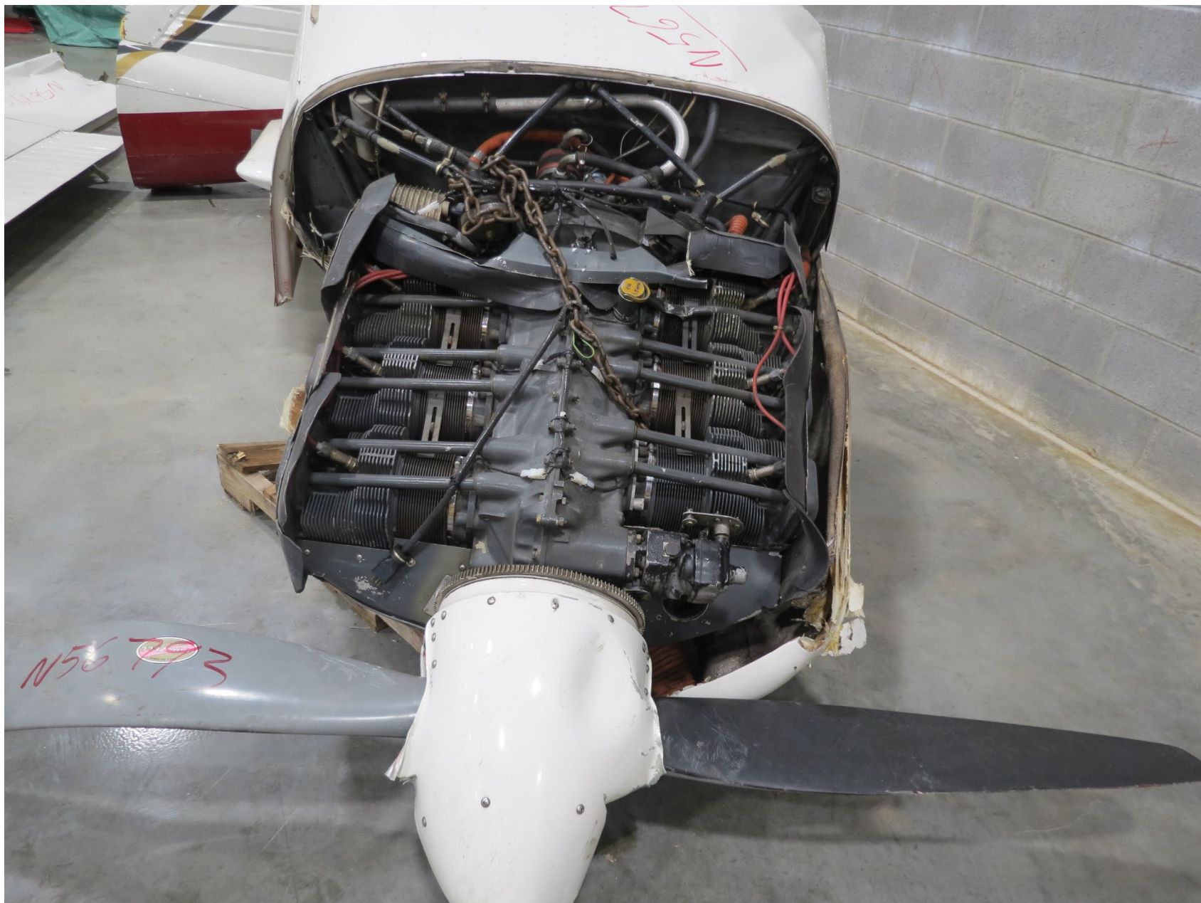
Photo 9 – View of the top of the engine during the examination (courtesy of Lycoming Engines).
