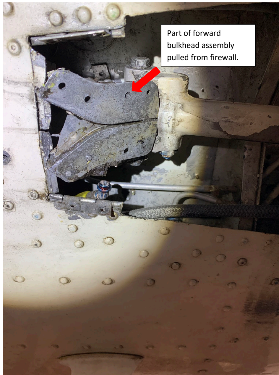
Photo 2 - Part of bulkhead assembly pulled from firewall
