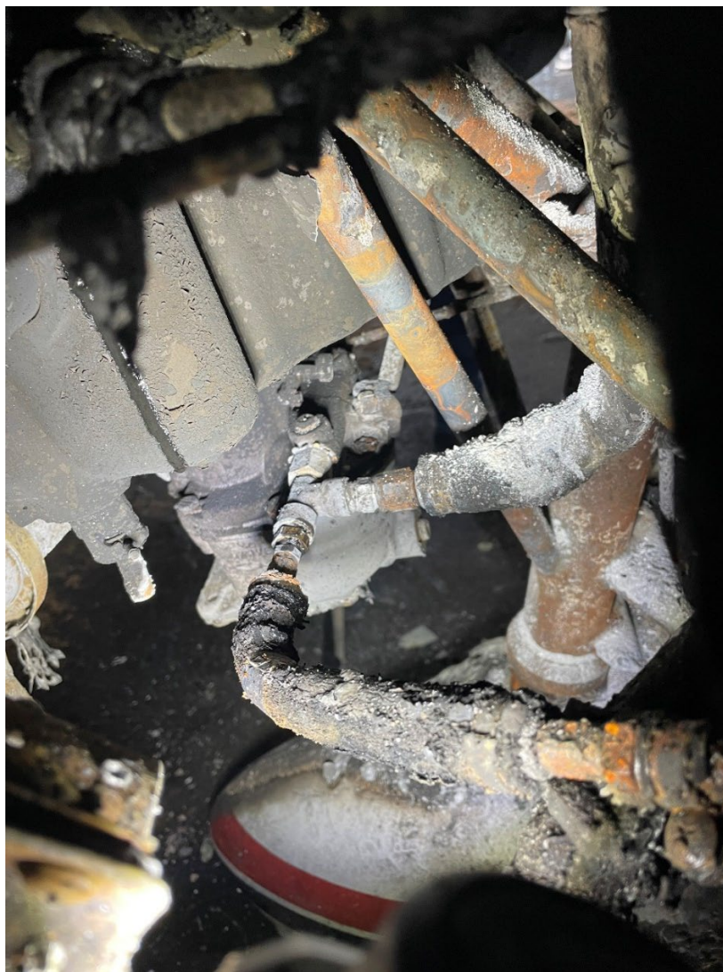
Photograph 5 – Carburetor Fuel Line (Courtesy of Federal Aviation Administration)
