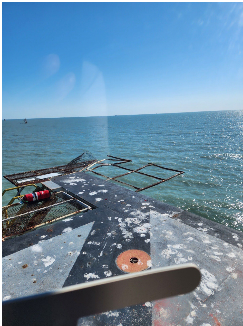
Photo 2 – Platform skirting damage (Source: Rotorcraft Leasing Company)
