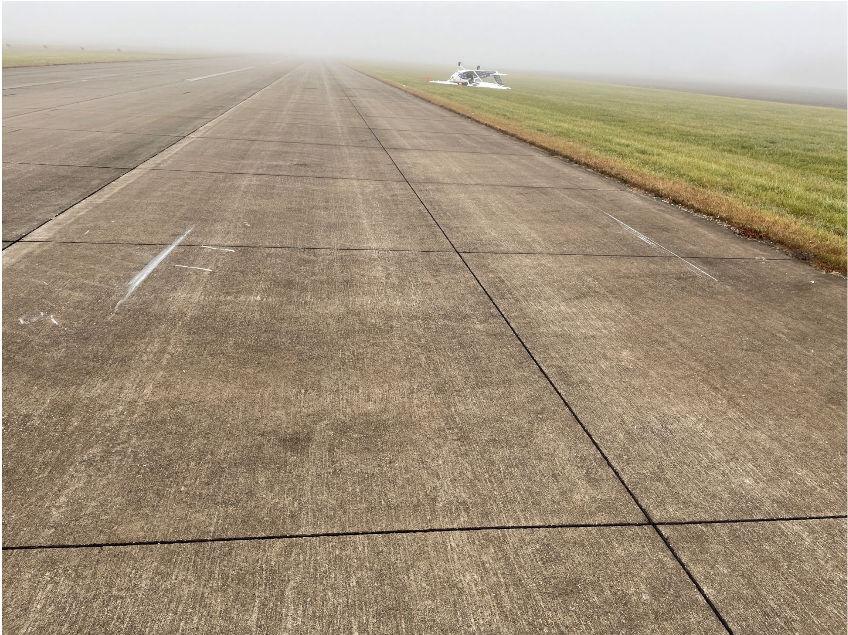
Photo 1 – Runway impact and propeller strikes (Source: Federal Aviation Administration)
