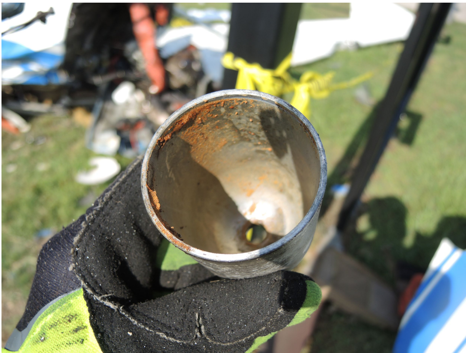
Photograph 11 - Debris in fuel strainer bowl
