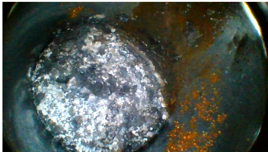
Figure 4. Cylinder #3 rust along piston head and walls.
