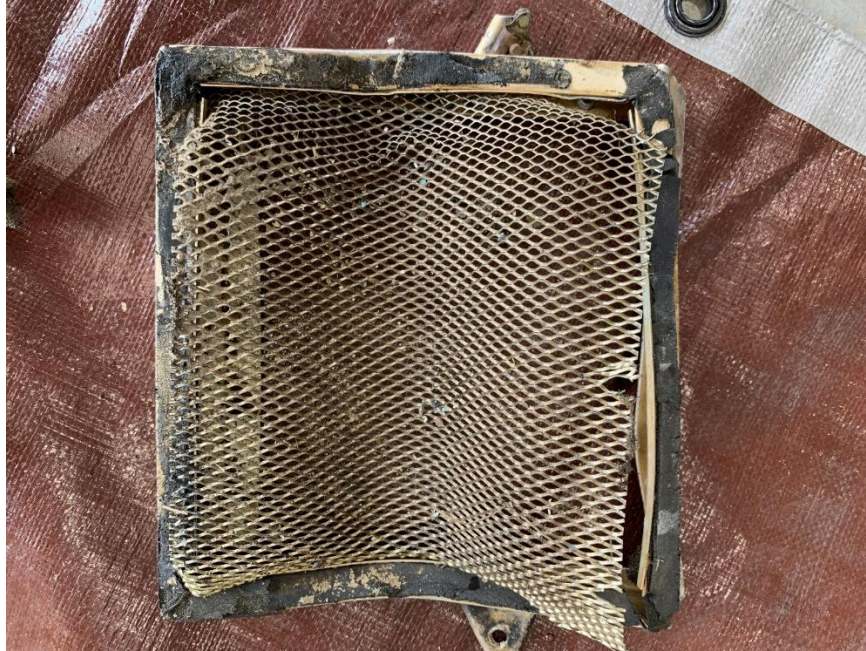
Figure 10. Engine induction filter box and gasket.
