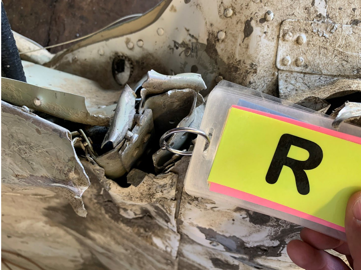
Right rear spar attach structure
