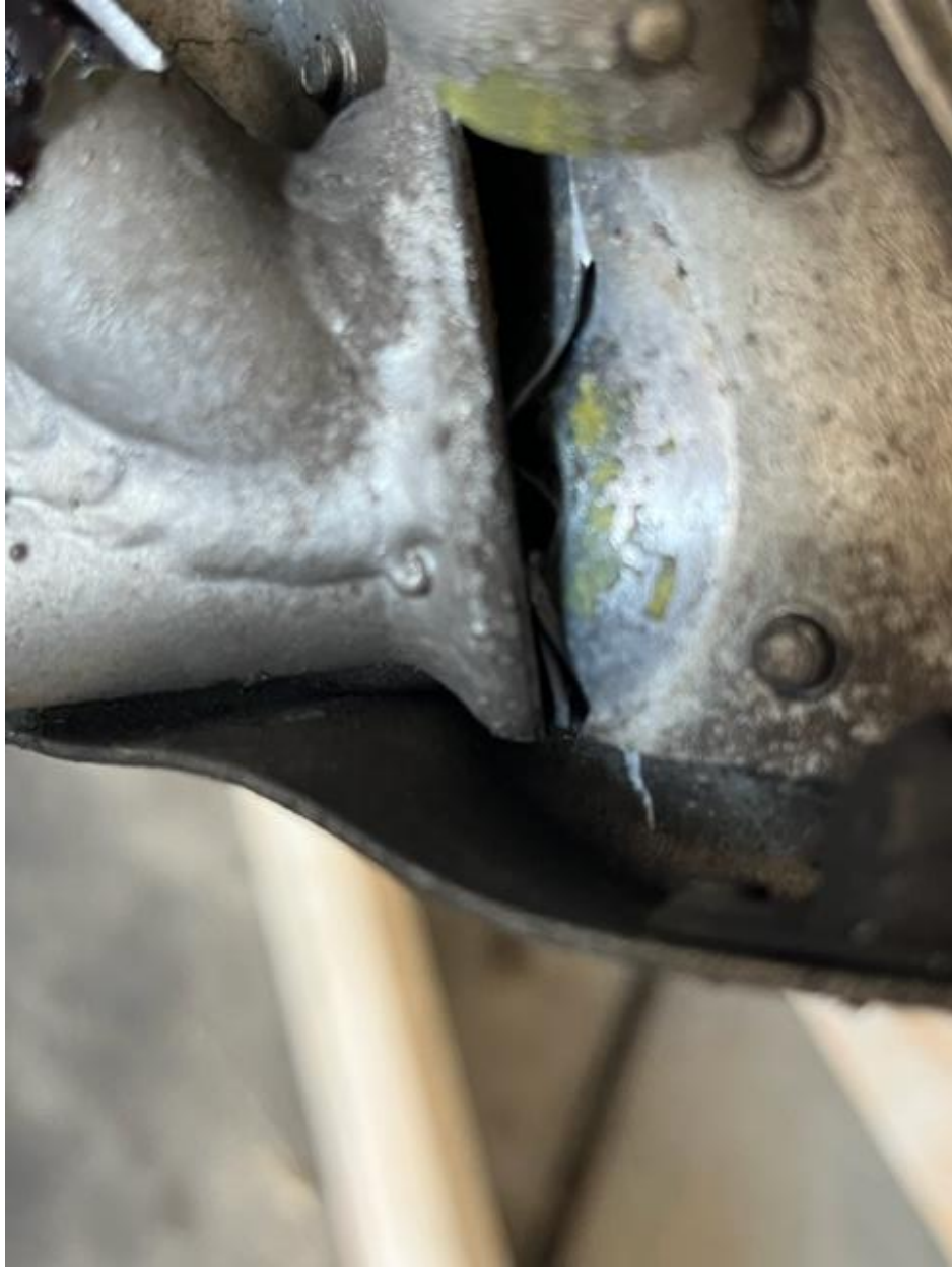
Photo 3: Lower Firewall Structure
