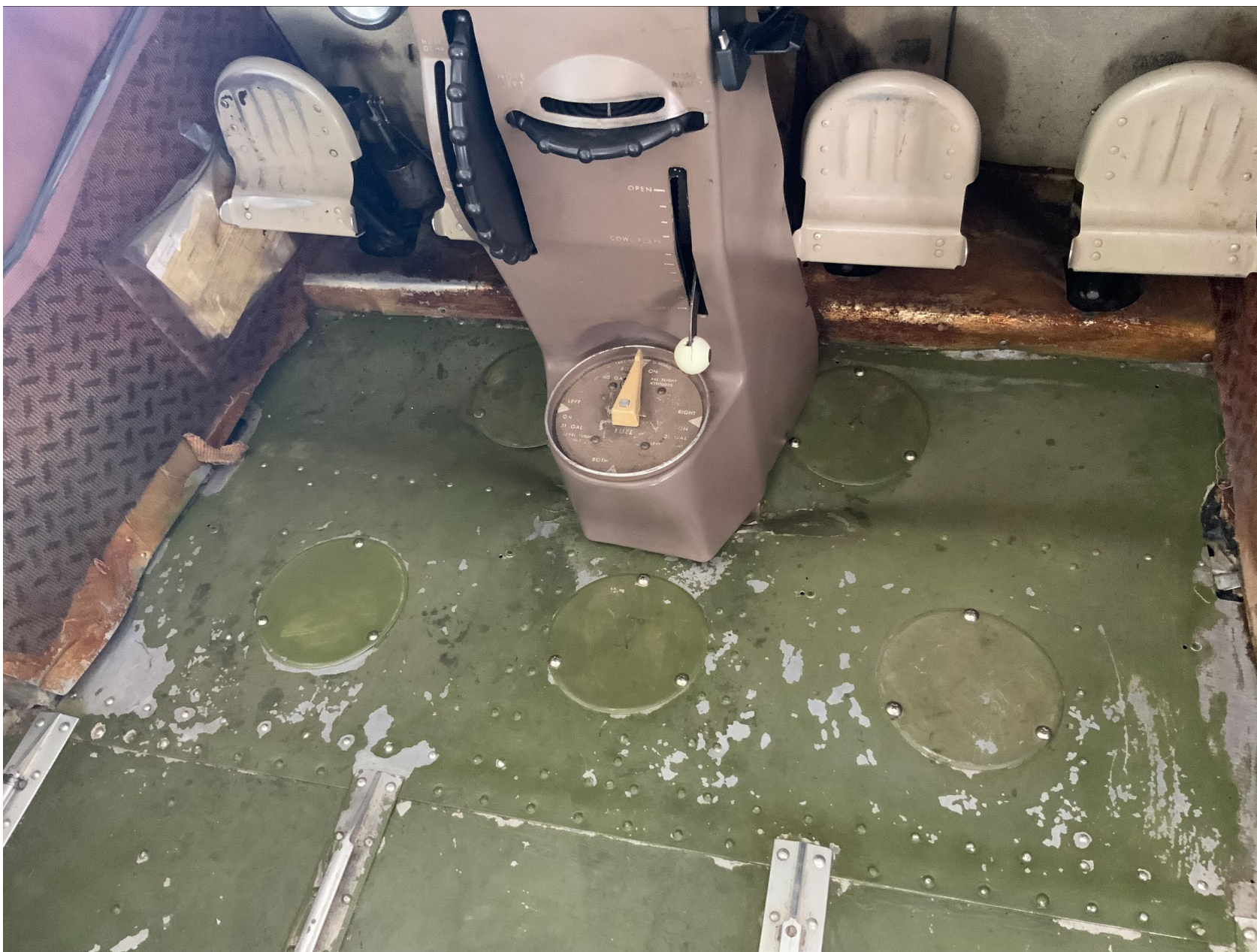
Photo 2 – Floorboard buckled (Courtesy of FAA)
