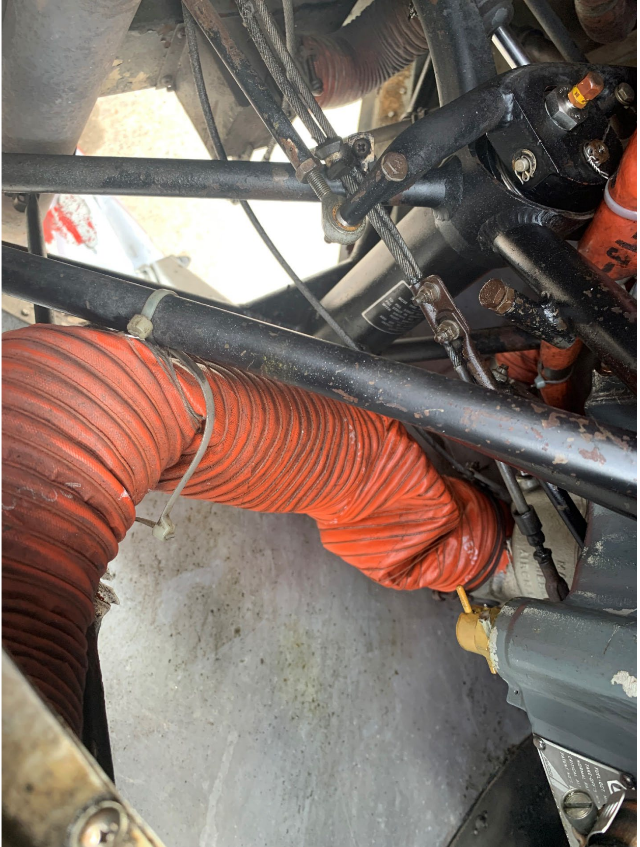
Figure 2: View of collapsed induction tube.
