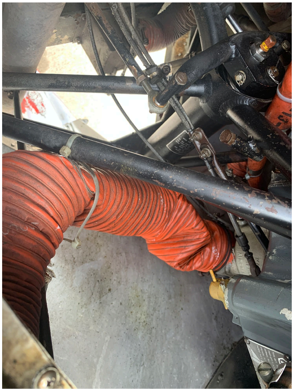
Photo 2 – View of partially collapsed induction tube (NTSB Photo)
